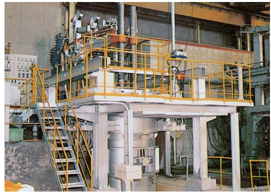
取鍋精錬炉 Ladle Furnace
